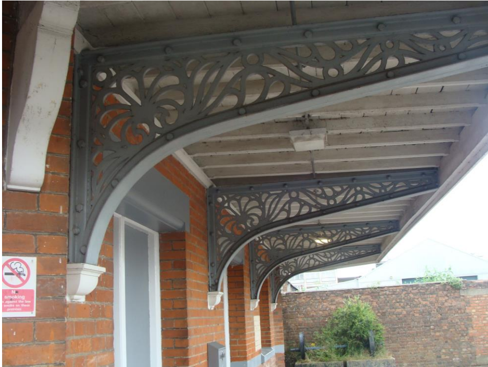
Picture 27. Typical late 19th/early 20 th century metal railway architectural brackets. Station building, London Road.
