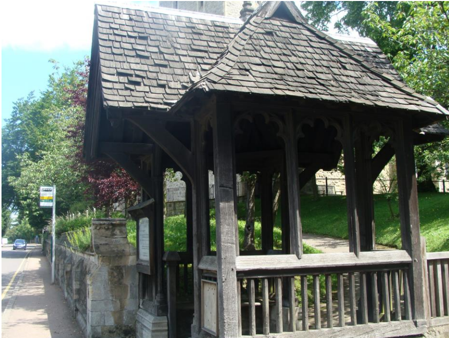
Picture 20. Lych Gate at Church of All Saints, of oak construction. Shingle roof and old bench seats,
