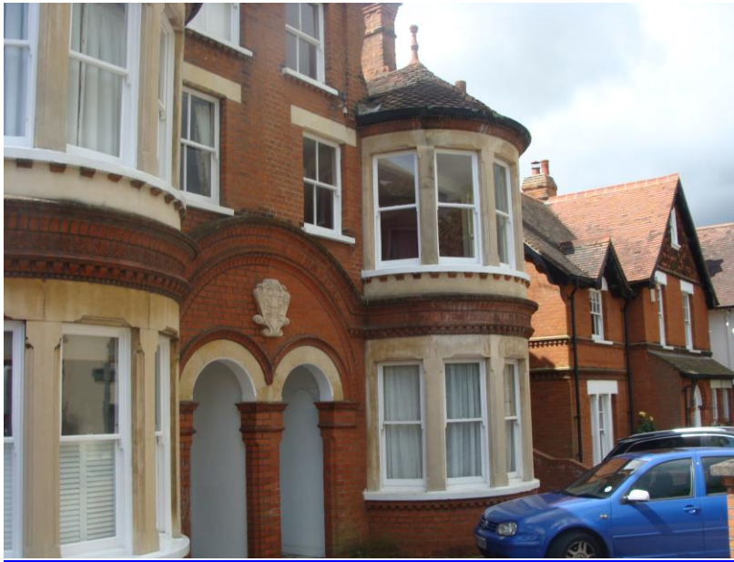
Picture 30. Nos.32-34 Grange Road, part of the street proposed to be included in an extended Conservation Area.
