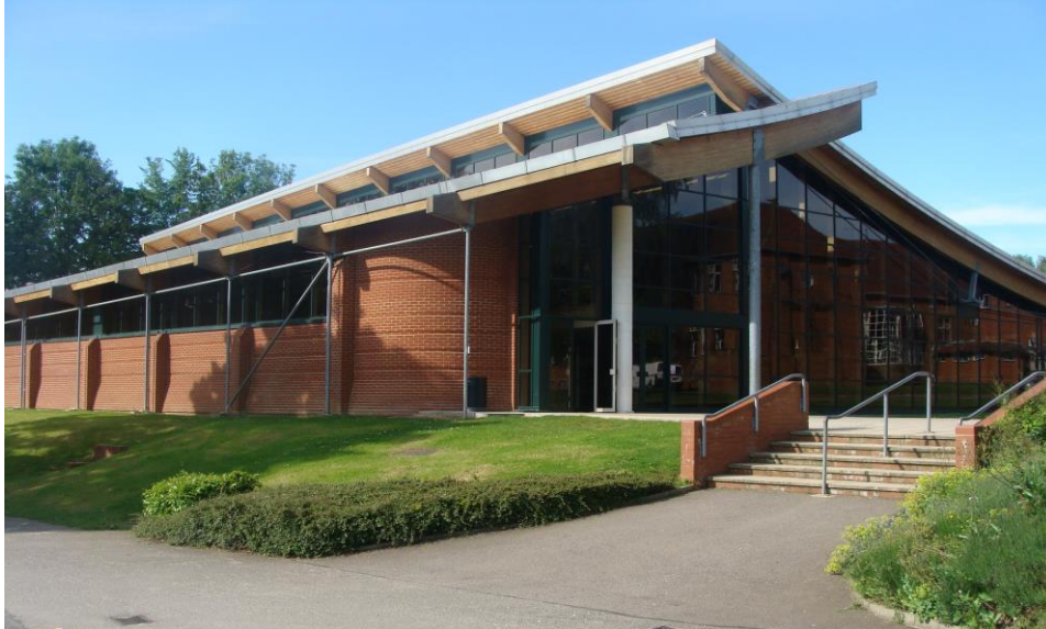
Picture 168. The simplicity and elegance of this contemporary building at Bishop's Stortford College adds to the range and diversity of quality buildings on the campus.
