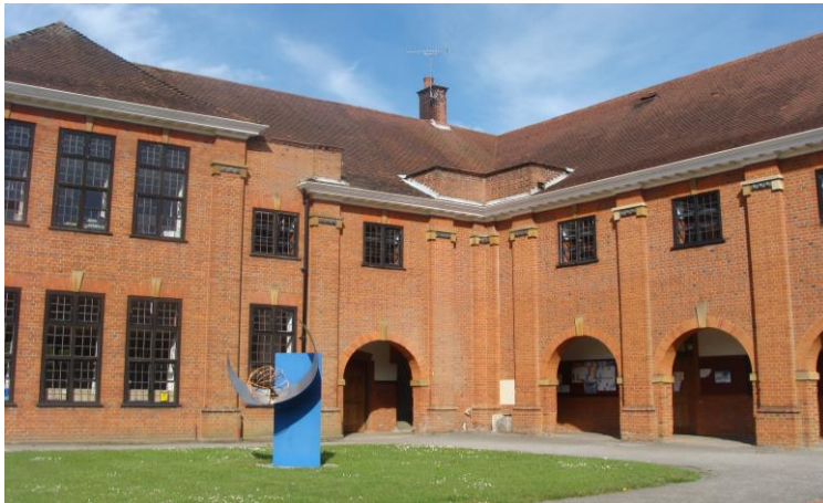
Picture 9. College building Maze Green Road dating from the early 20 th century.
