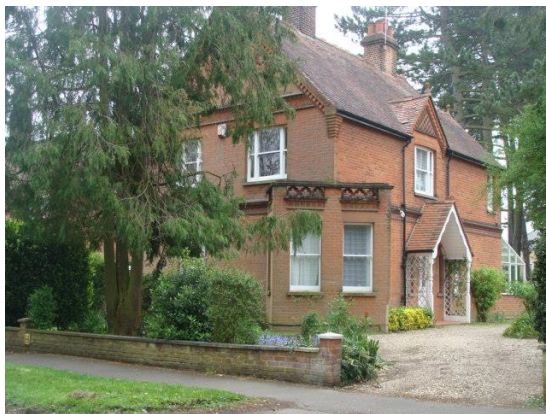
Picture 31. No. 66 Warwick Road with unusual diagonally aligned windows to front elevation, one of three such examples in the street.
