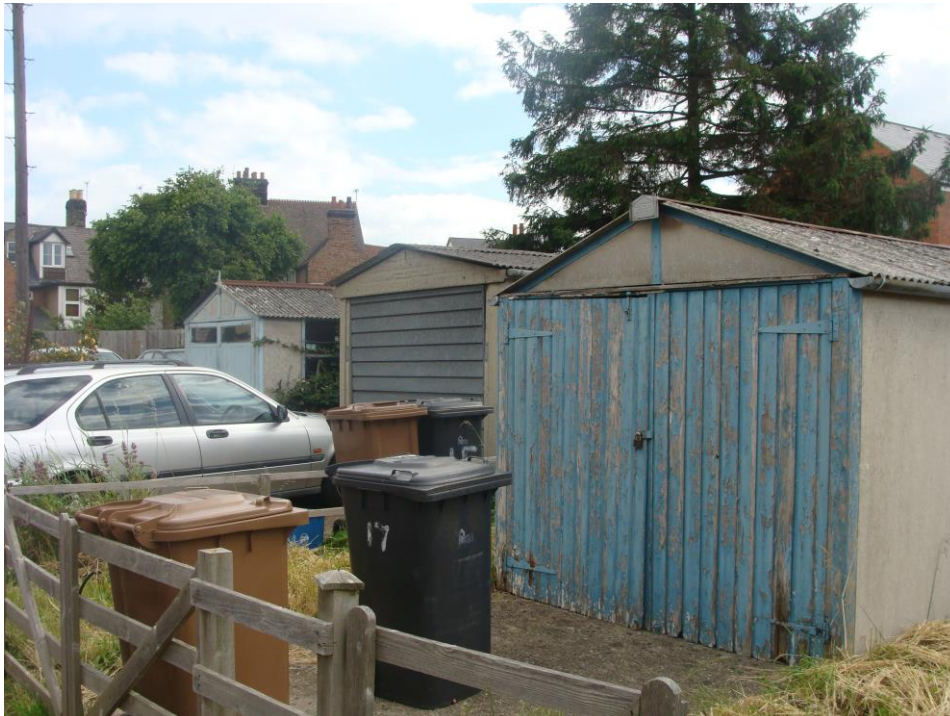
Picture 327. Garaging of a temporary nature associated with Crown Terrace adjacent to EHDC surface car park. Views relating to the future of this whole area are sought.
