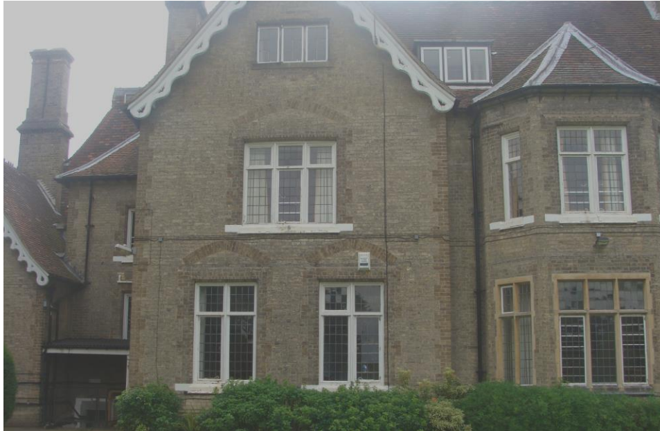
Picture 22. Thames House, old block. Good quality 'curtilage listed' 19 th century accommodation on the Hockerill Anglo- European College campus.
