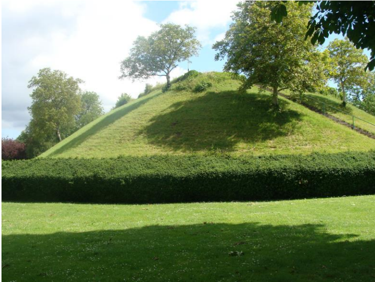
Picture 413. Waytemore Castle of significant visual historic and archaeological importance. A careful assessment is suggested particularly in relation to security, erosion and vegetation.
