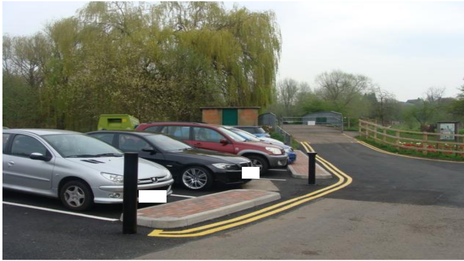
Picture 56. The metal barriers of previous picture now replaced with raised surface and bollards.
