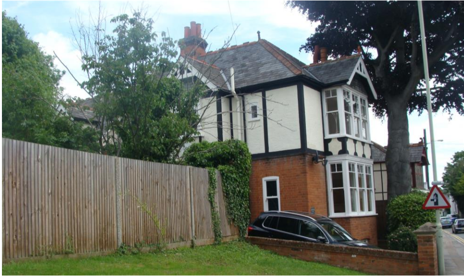
Picture 12. No. 30 Hadham Road, Oakbeam. Two storey house dating from early 20 th century. Selected architectural features are worthy of additional protection.
