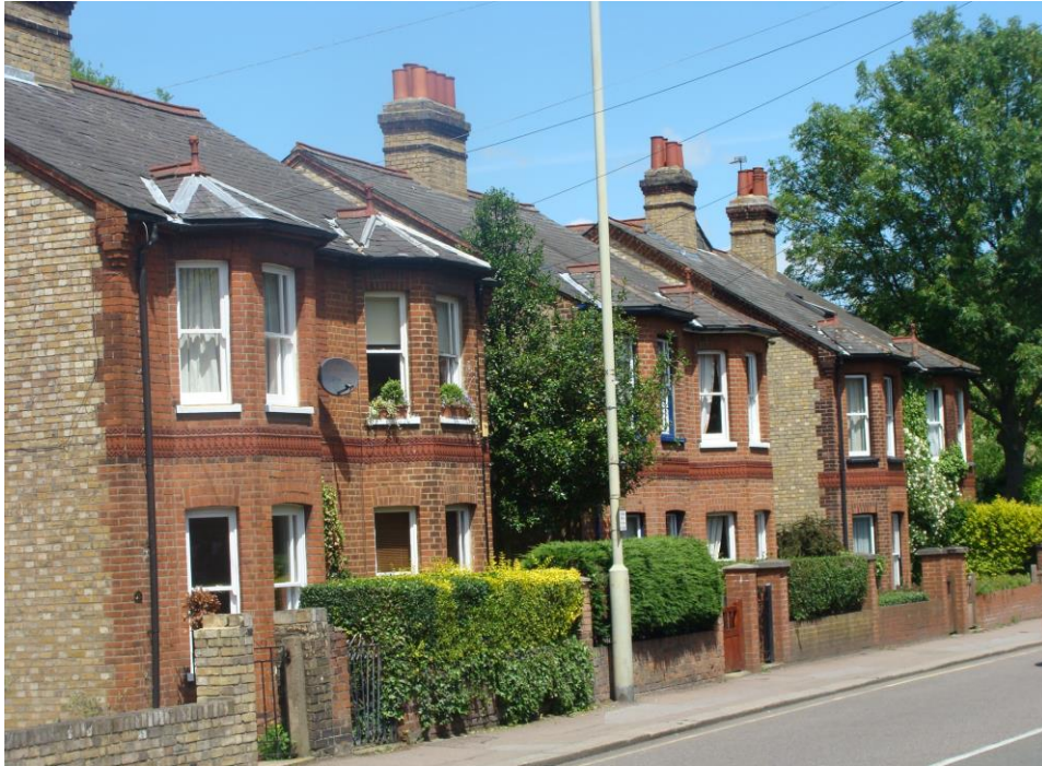
Picture 25. Nos. 25-35 Stansted Road. Repetitive architectural detailing adds to their individual quality and quality as a group.
